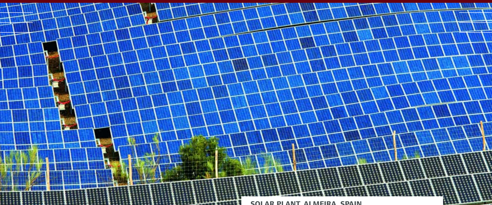
SOLAR PLANT, ALMEIRA, SPAIN
